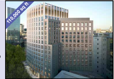
Wedge House SE1
